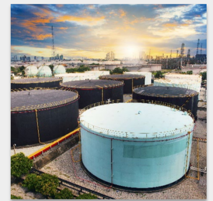
Monitoring of industrial plants
