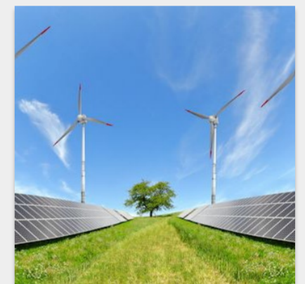
Intelligent control of power grids
